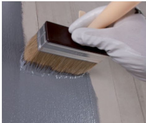
Application of Eco Prim Grip Plus on concrete by brush
