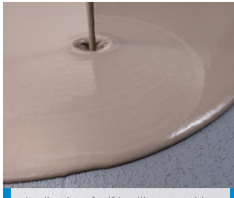
Application of self-levelling smoothing compound on dry Eco Prim Grip Plus on old floor
