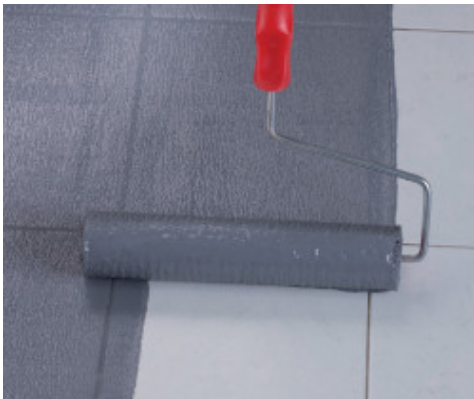
Application of Eco Prim Grip Plus by roller on existing porcelain tiles
